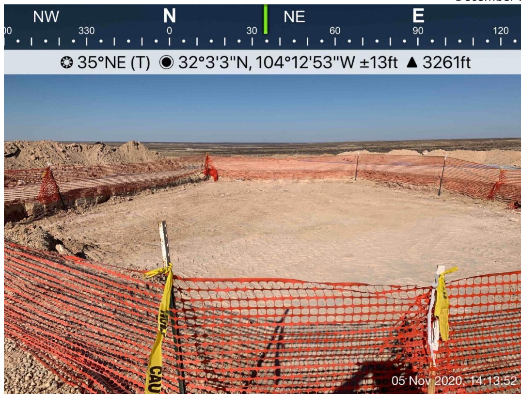
Diesel Spill Area Excavation Viewing Northeast, November 5, 2020
