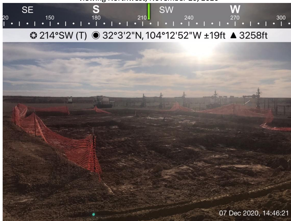
Additional Soil Removed from the Sidewall (N-SW) and Bottom C'-6 from the Oil Based Mud Spill Excavation viewing Southwest, December 7, 2020
