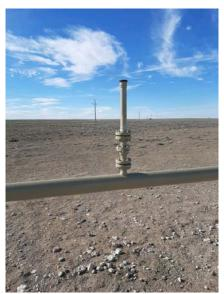
Figure 1: Release point of blowdown emissions
