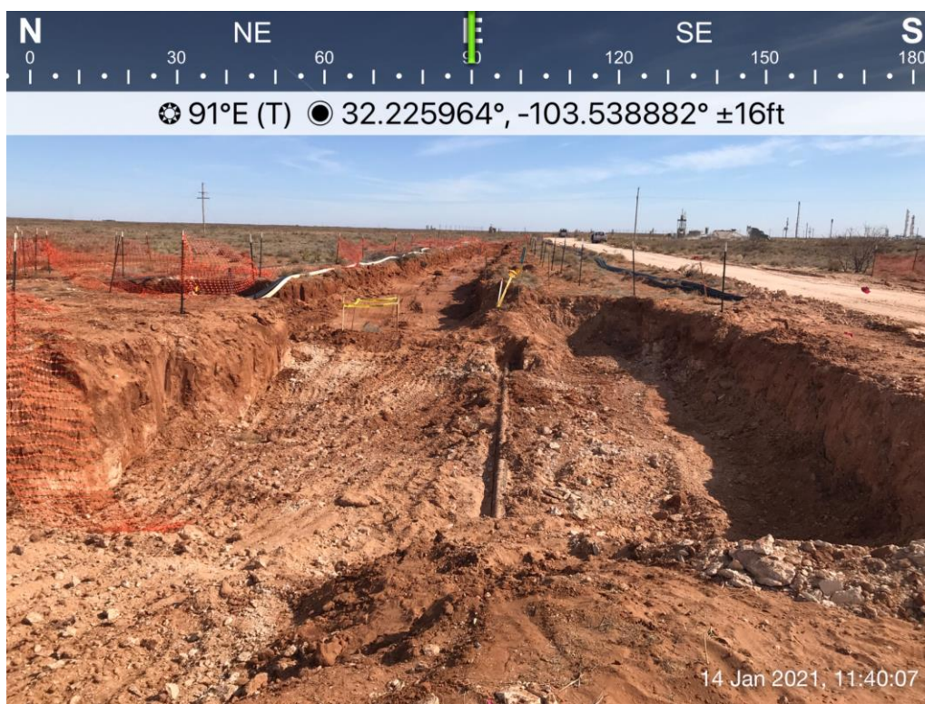
View East, area of Bottom Holes (76-88)
