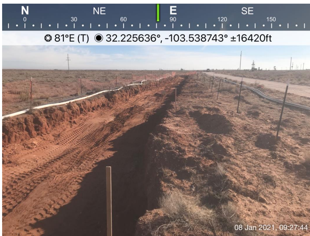
View East, area of Bottom Holes (39-64)
