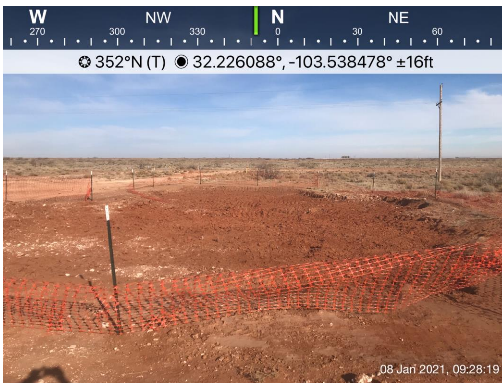
View North, areas of Bottom Holes (1-22)
