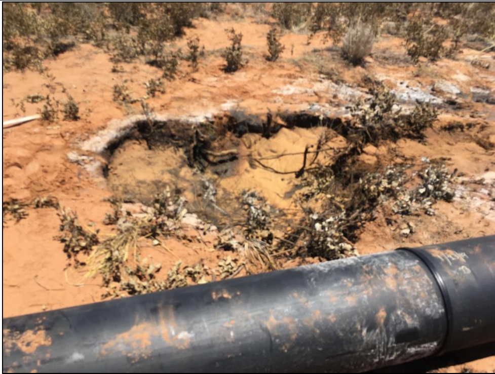
PHOTO 1: View of Release Origin, facing East. 6/07/2019
