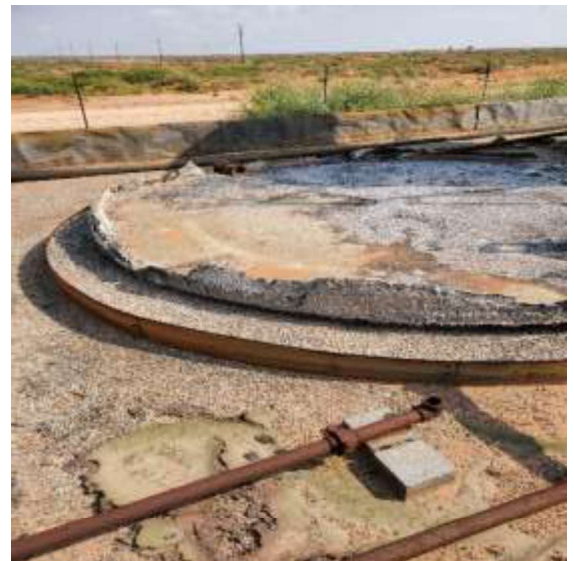
Remnant of tank bottom post lightning strike
