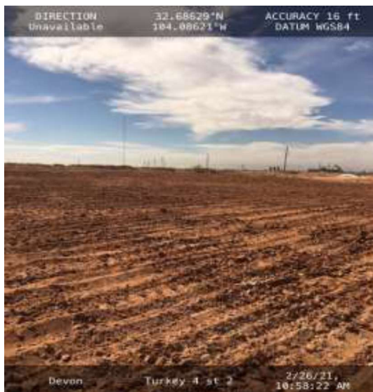
Pad reclaimed 4' of topsoil re-seeded
