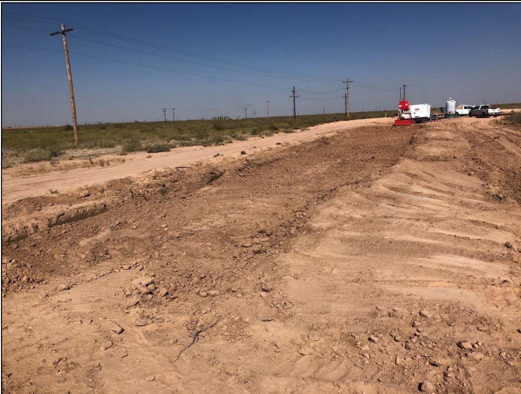
PHOTO 6: View of Excavation around HA-1 / HA-2, facing north. 12/01/2020
