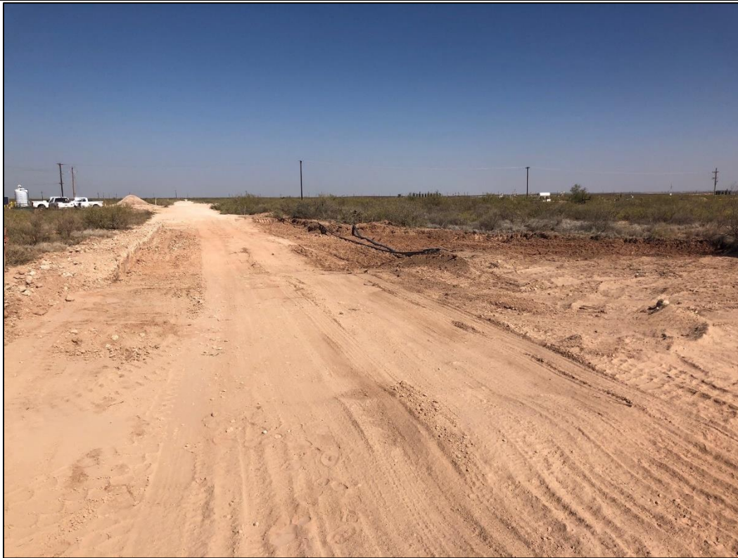
PHOTO 4: View of Excavation around HA-4 / HA-5, facing north. 12/01/2020
