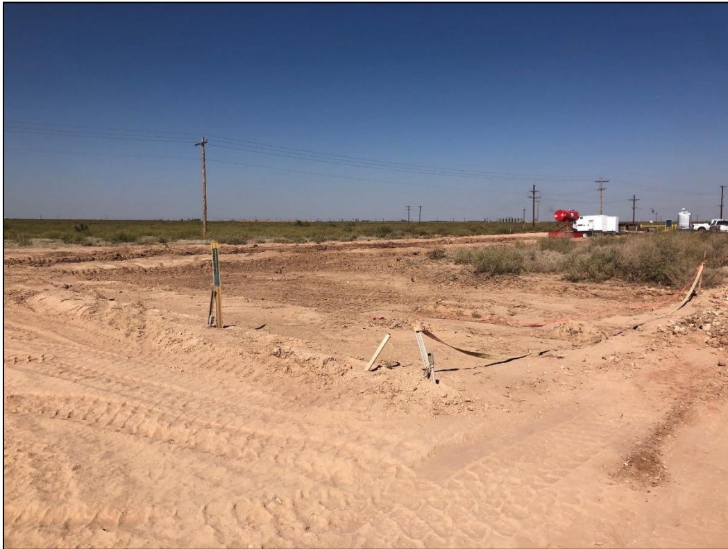
PHOTO 5: View of Excavation around HA-3, facing northwest. 12/01/2020
