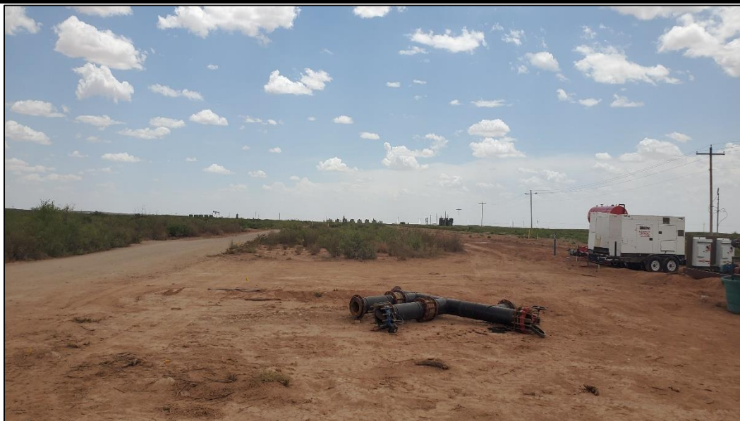
PHOTO 1: View of Release area, facing south. 7/21/2020
