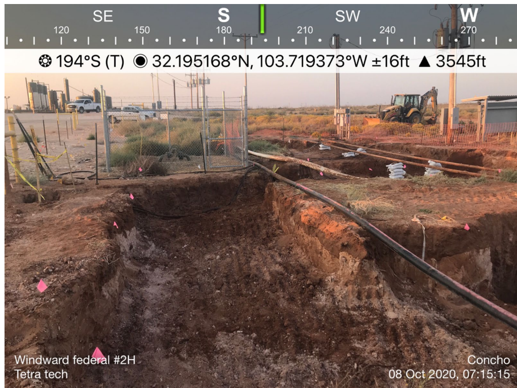
South View of Remediation Activities
