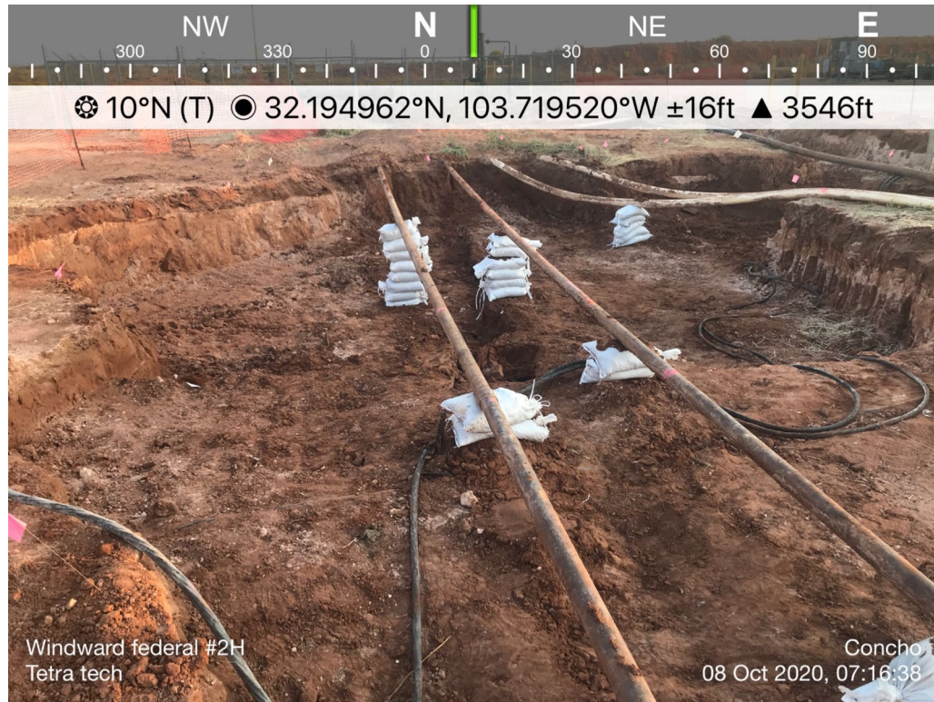
North View of Remediation Activities
