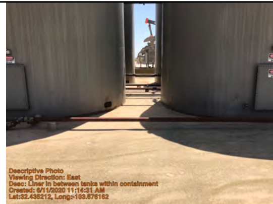
Liner in between tanks within containment
