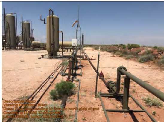
Flow lines leading to flare on north side of pad
