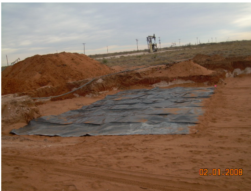
Photograph No. 9 – Installation of 40-mil liner over northern deep excavation.
