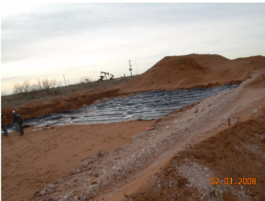
Photograph No. 10 – Installation of 40-mil liner over central deep excavation.
