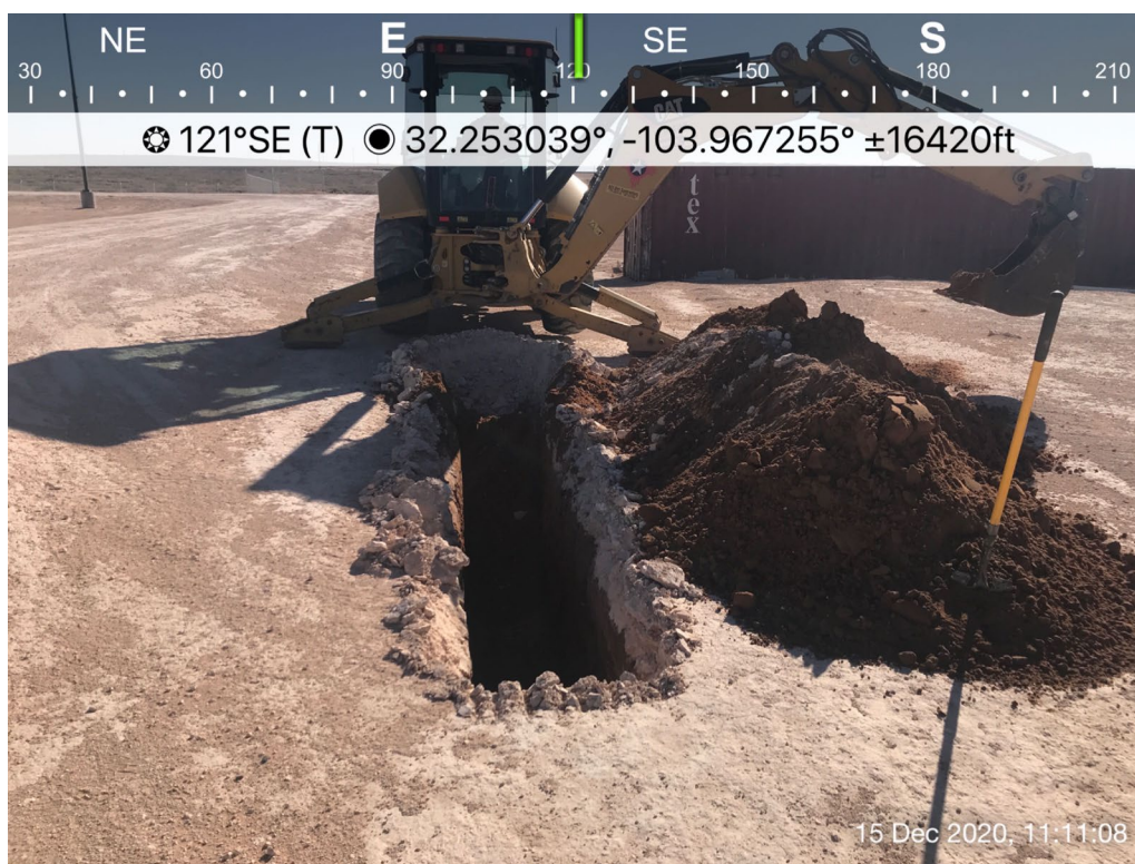
View of Trenching Activities – View Southeast
