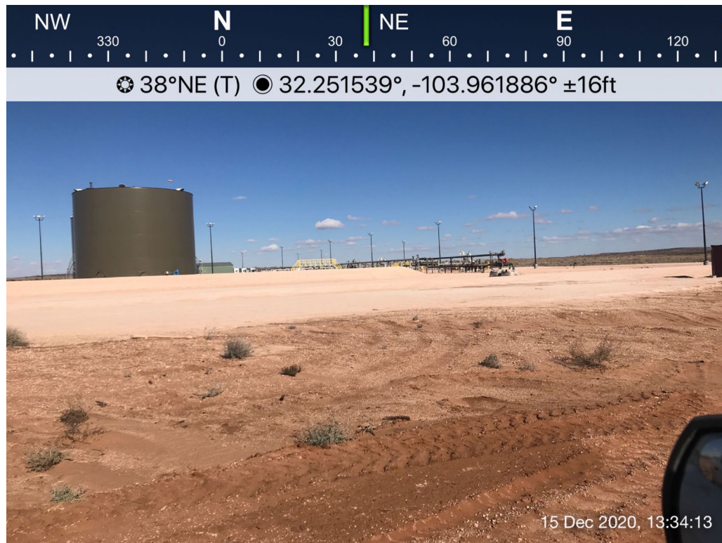
View of Release and Pad Area – View Northeast
