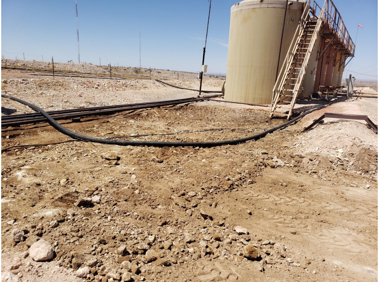
REMOVAL OF 1 FT OF CONTANMATED SOIL
