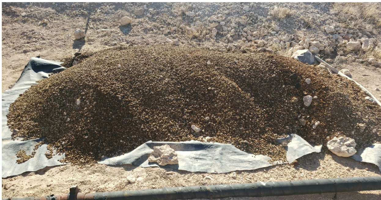
ENRON STATE BATTERY CLEANUP AROUND KNOCKOUT OF 1 FT
