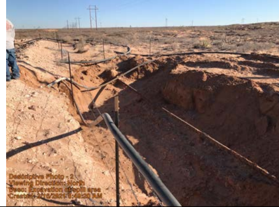
Excavation of spill area
