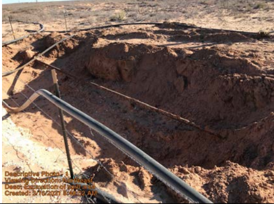
Excavation of spill area
