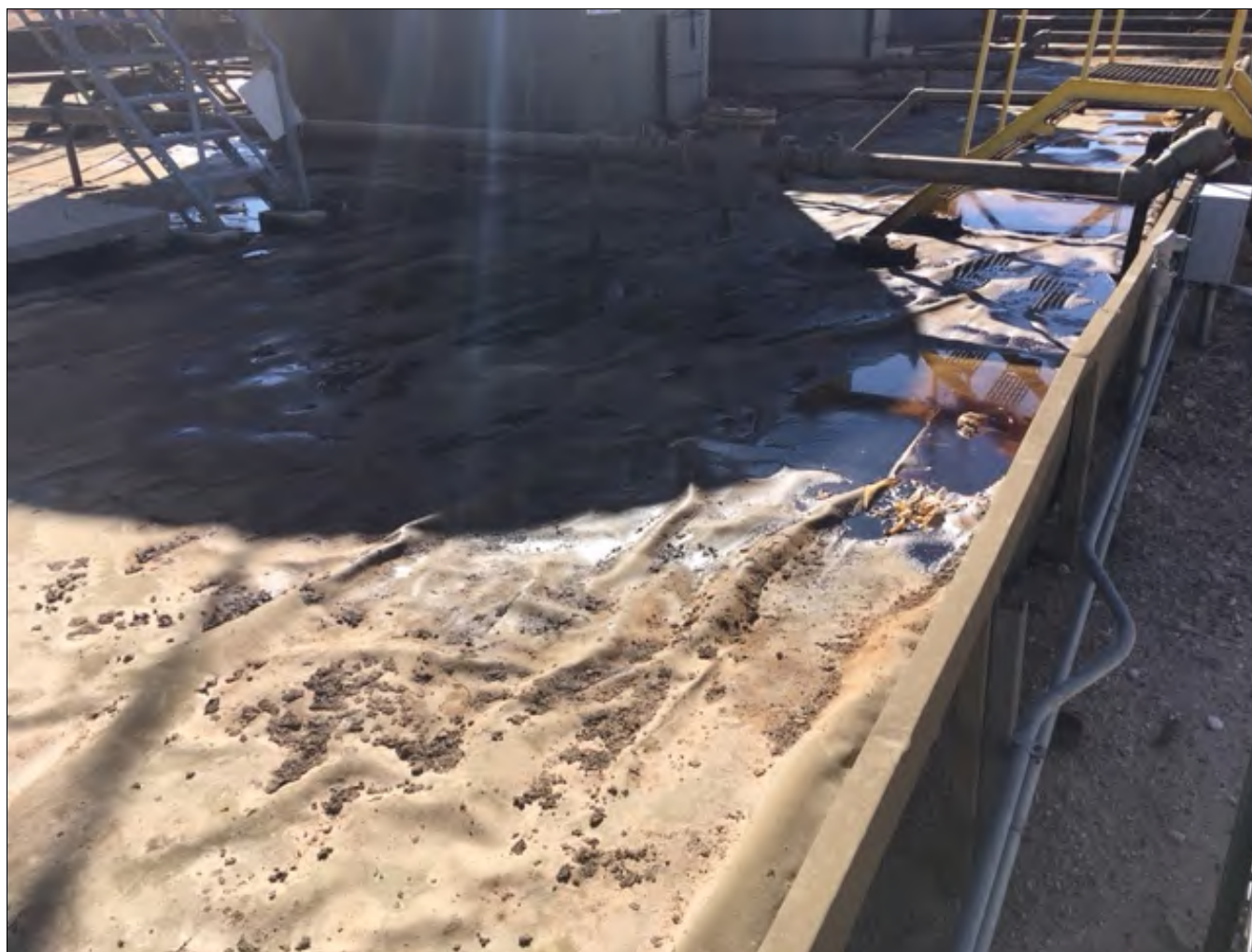
View of lined tank battery containment and liner hole during soil sampling activities.
