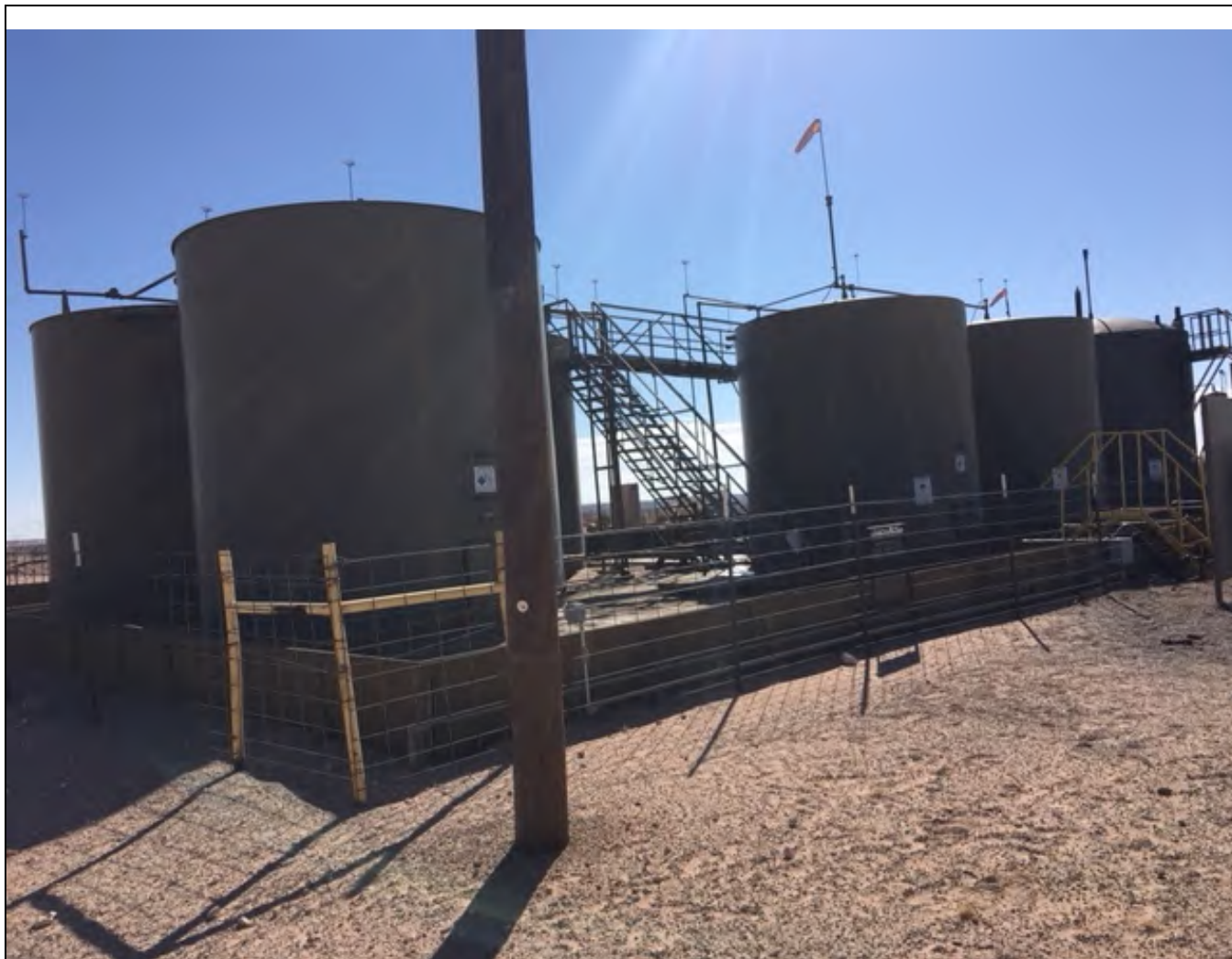
Western view of lined tank battery containment.
