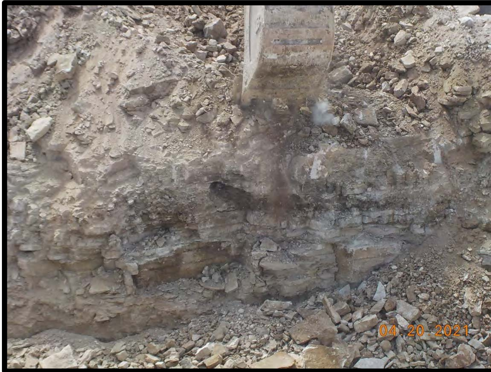
PHOTOGRAPH NO. 9 – A view of the rocky conditions observed within the pipeline area during assessment activities on April 20, 2021.
