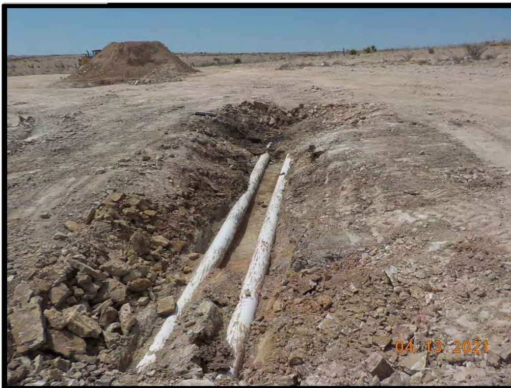
PHOTOGRAPH NO. 5 – A view two out-of-service PVC lines upon exposure. The view is towards the northwest.
