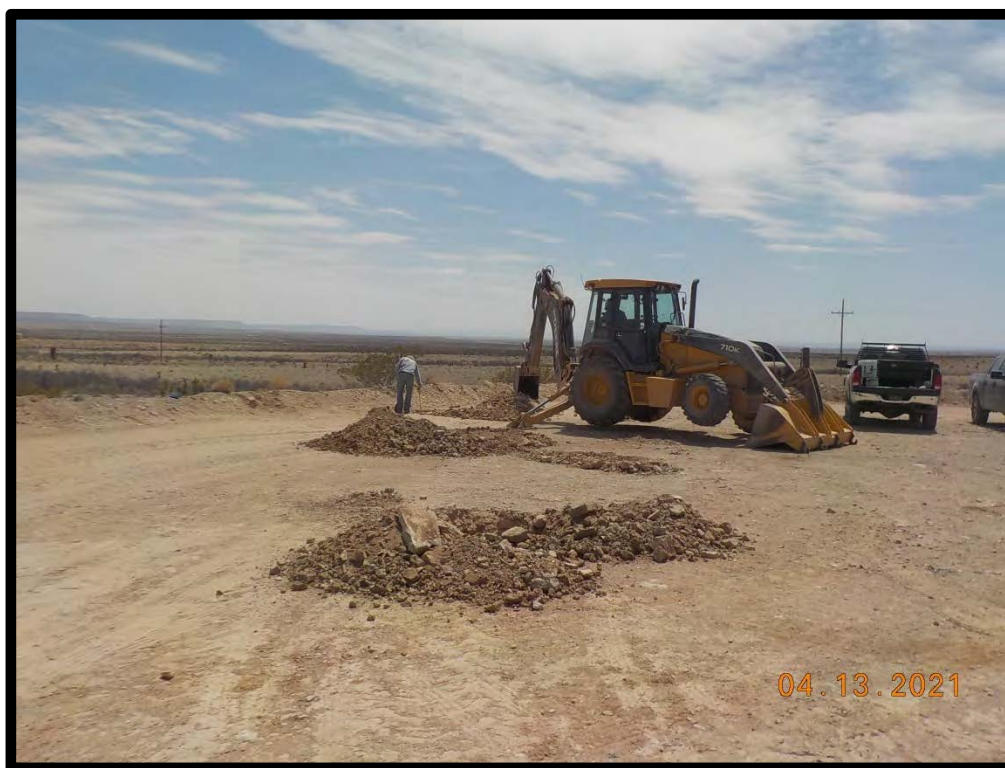
PHOTOGRAPH NO. 3 – A view of the additional assessment activities in facility pad area. In the view test hole excavations “TH-S.4”, “TH-S.5” and “TH-S.6” are visible. The view is towards the south.
