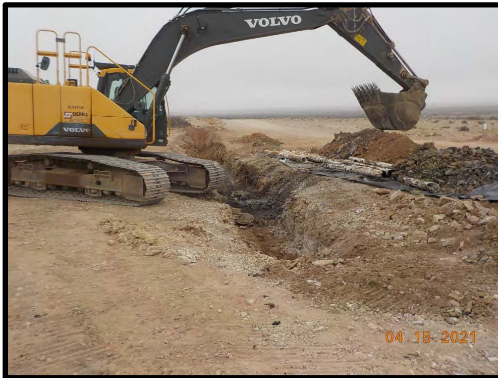
PHOTOGRAPH NO. 7 – A view of the pipeline area during the removal of the out-of-service PVC lines. The view is towards the southeast.
