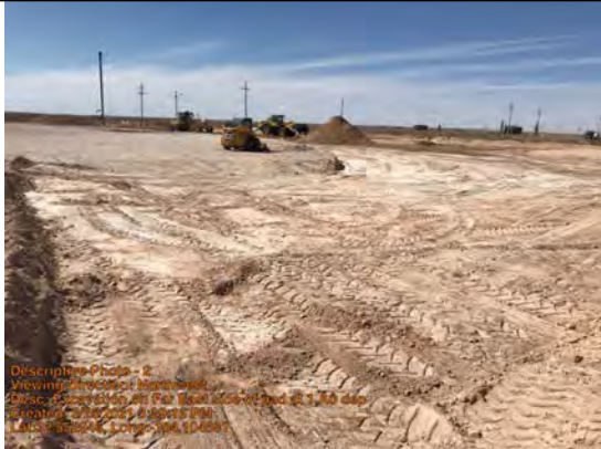
Excavation on Far East side of pad at 1' depth
