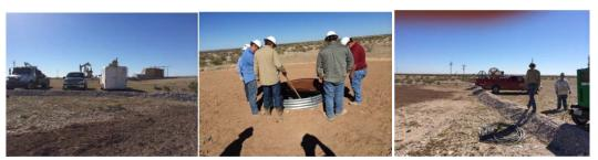
c. 9:50-am Excavation of the 6" PVC lines north of the Johnson BE battery begins. Excavation Sloped to 30% and sampled for hazardous atmosphere. Cut made and valve installed under air.
