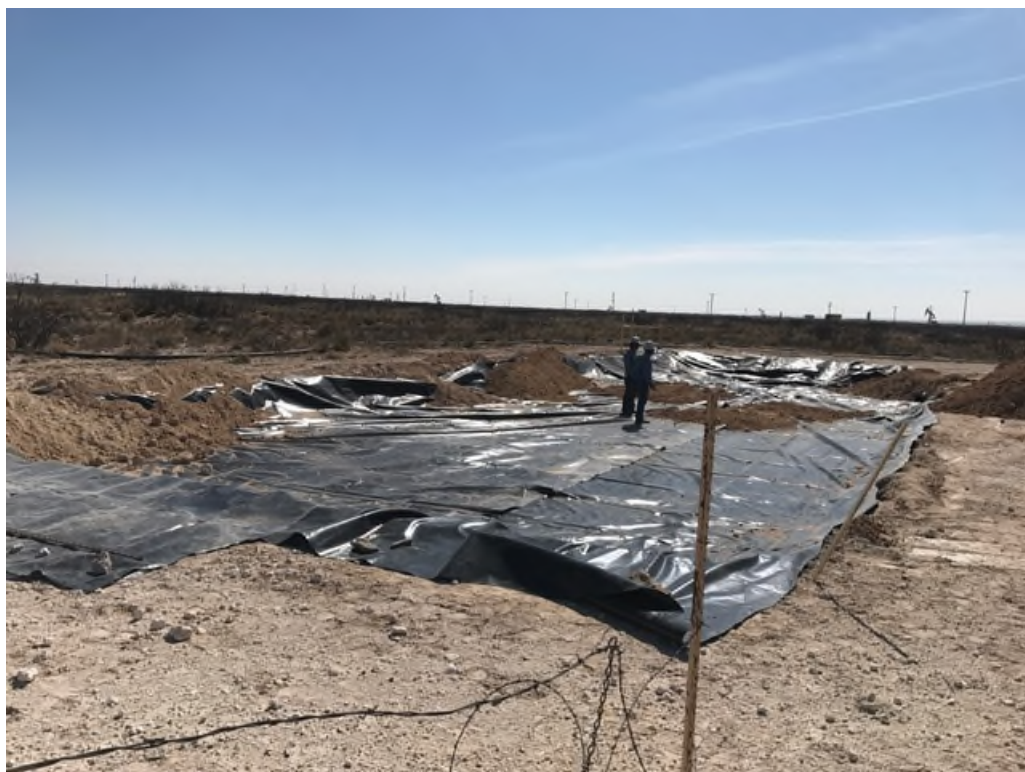
Area SP-5 and SP-4 Liner Installation – View to Southeast
