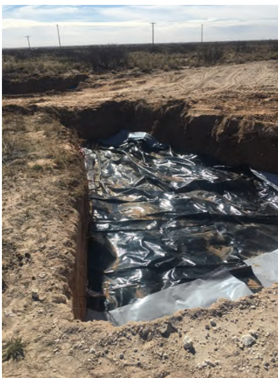
Area of SP-2 Liner Installation – View to South
