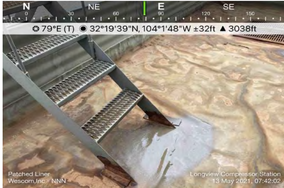
Patched Liner North of Tank F55472
