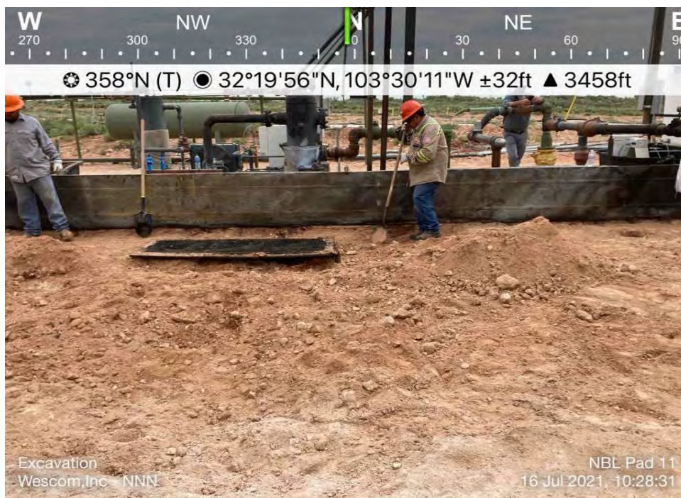
Excavation of Spill Area
