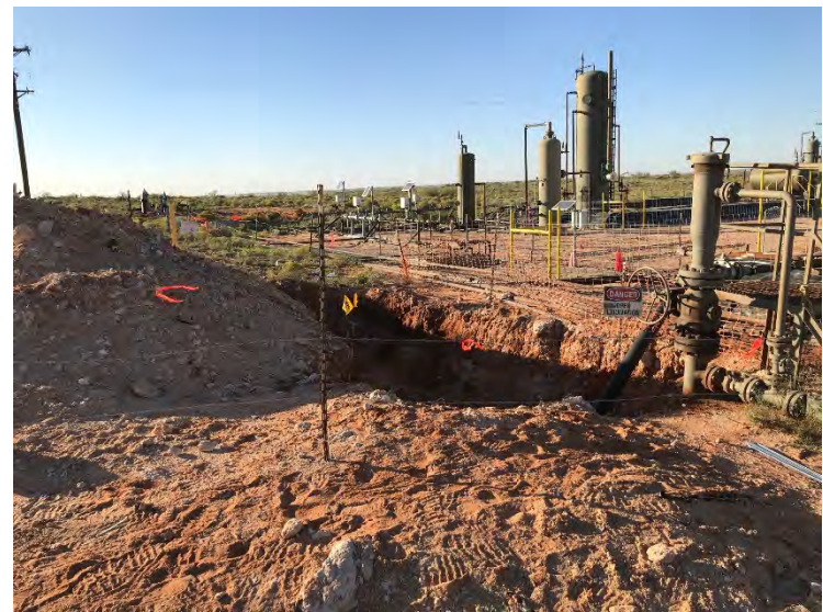
Photograph 12: View of open excavation (2RP-4398), facing northwest.
