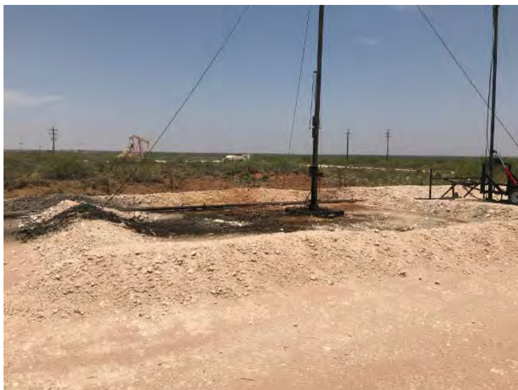
Photograph 5: View of release area (2RP-4775 and 2RP-4779), facing north.
