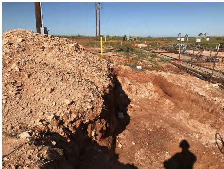
Photograph 11: View of open excavation (2RP-4398), facing west.
