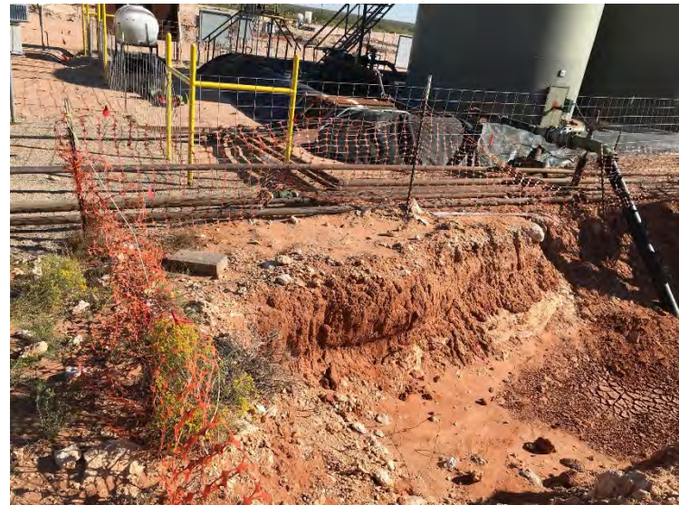
Photograph 10: View of open excavation (2RP-4398), facing north.
