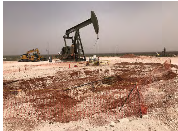
Photograph 4: View of excavation (2RP-2526), facing northeast.
