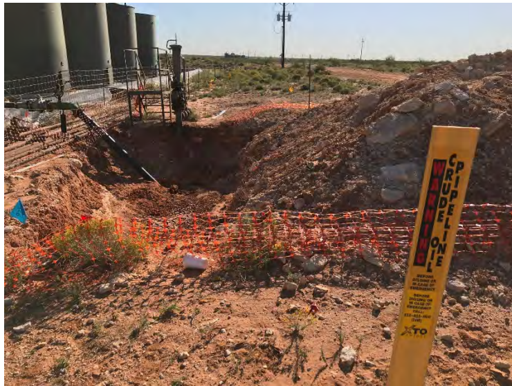
Photograph 9: View of open excavation (2RP-4398), facing east.
