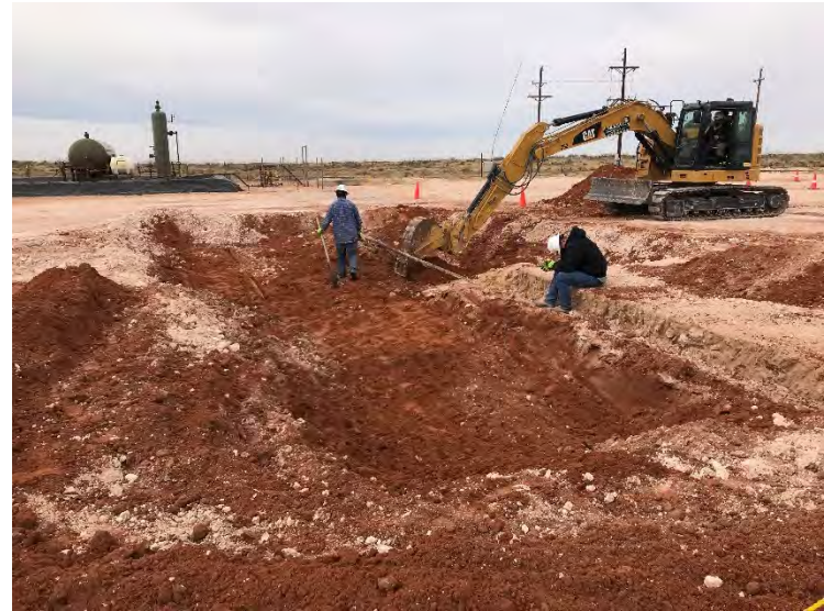
Photograph 2: View of excavation (2RP-2526), facing west.
