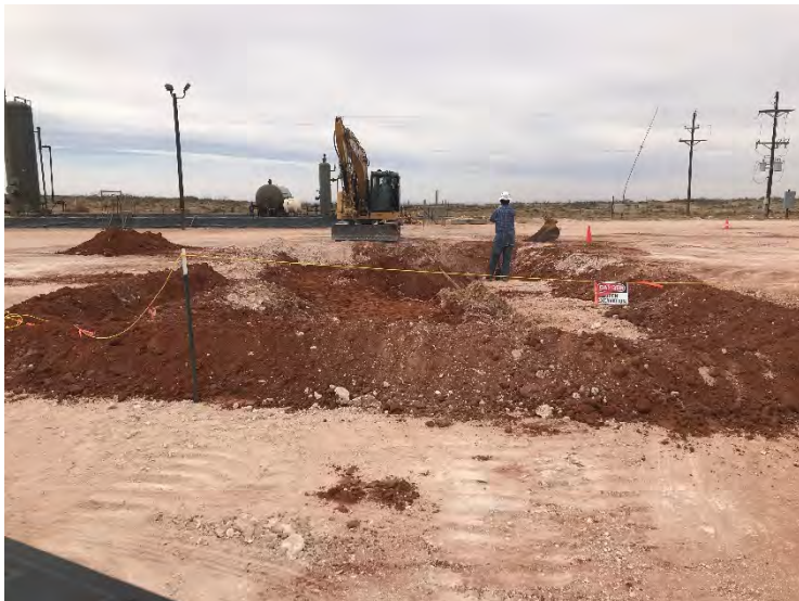
Photograph 3: View of excavation (2RP-2526), facing west.
