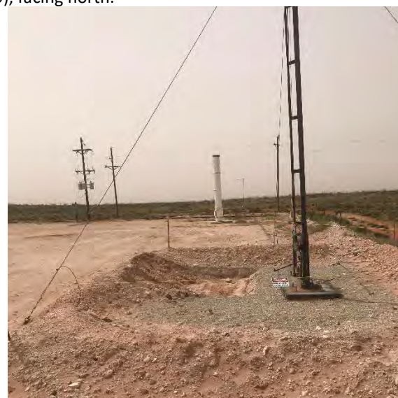
Photograph 8: View of release area and excavation (2RP-4775 and 2RP-4779), facing west.
