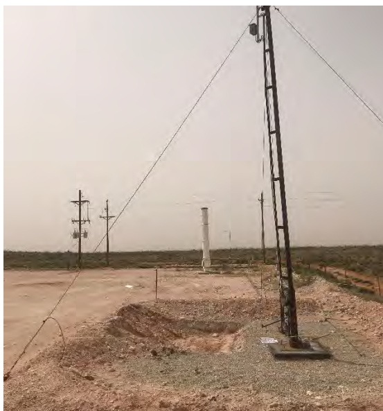
Photograph 7: View of release area and excavation (2RP-4775 and 2RP-4779), facing west.
