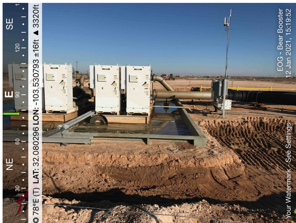
View of Remediation Activities – View East
