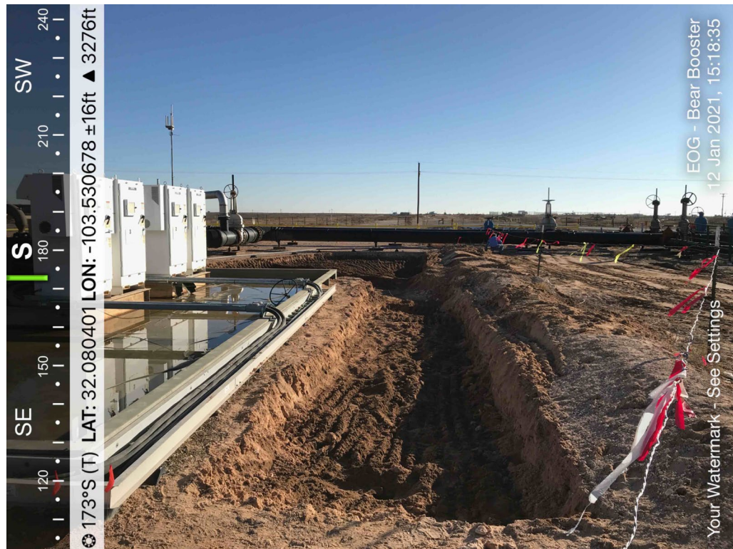
View of Remediation Activities – View South
