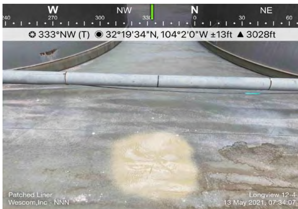
Liner Patched Between T-17441 and T-17442
