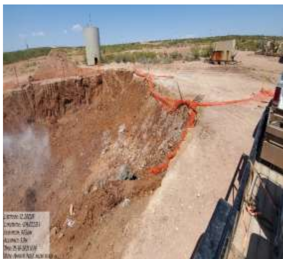
Application of Micro-blaze sidewalls
