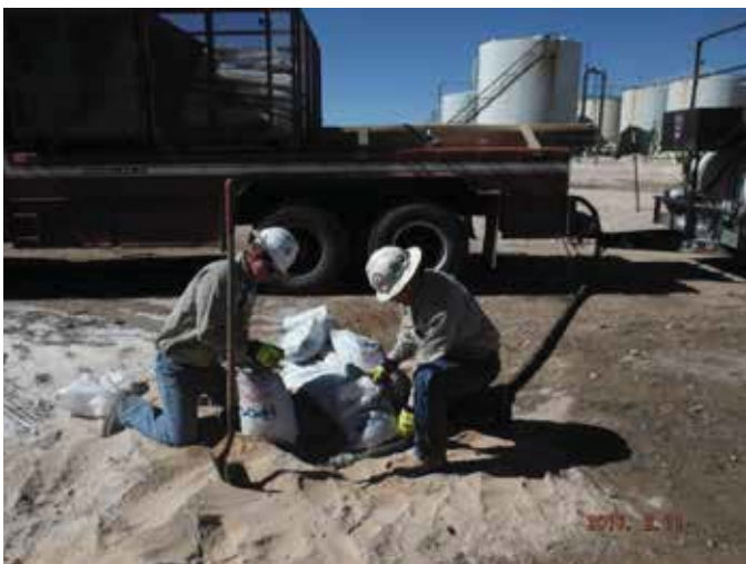
Plugging soil bore #2, facing west 2/11/16
