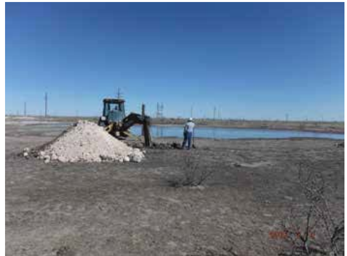
Installing vertical #2, facing north east 2/9/16
