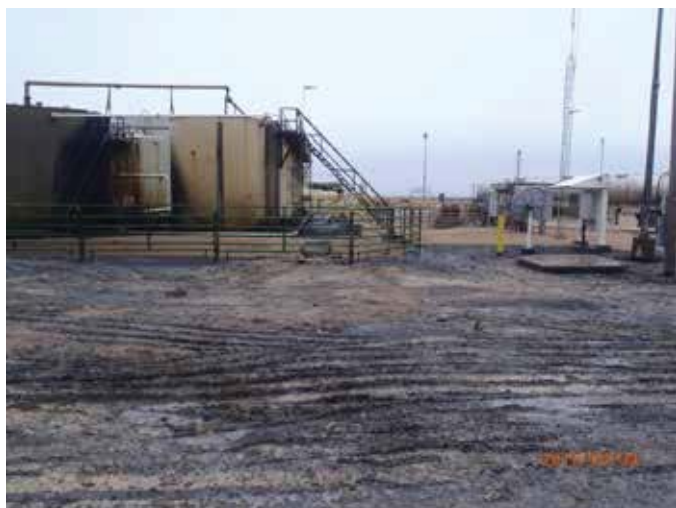
Initial release area, facing south 3/4/15
