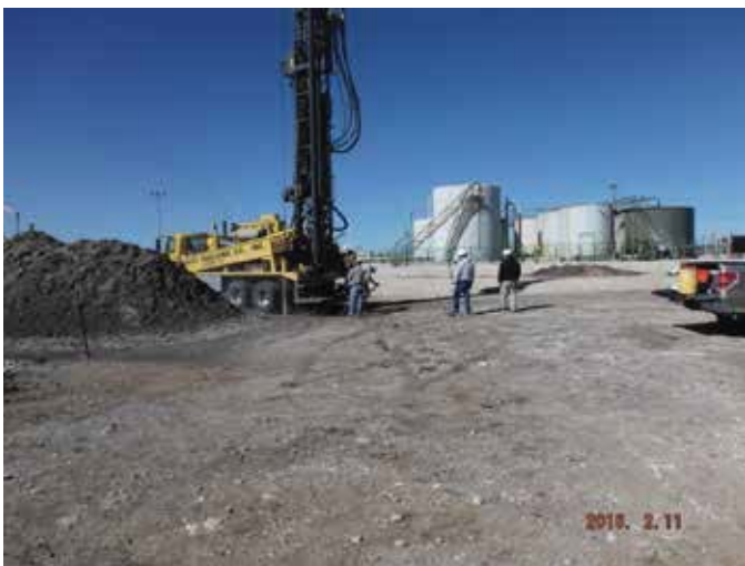
Installing soil bore #2, facing west 2/11/16
