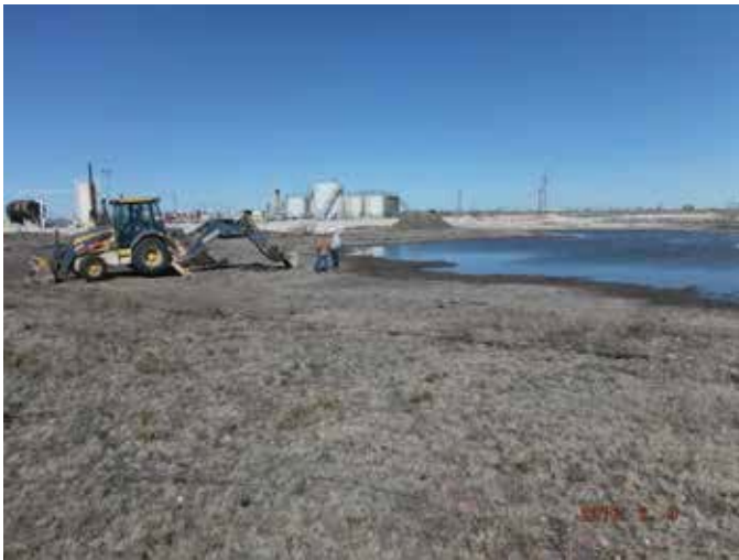
Installing vertical #1, facing north west 2/9/16
