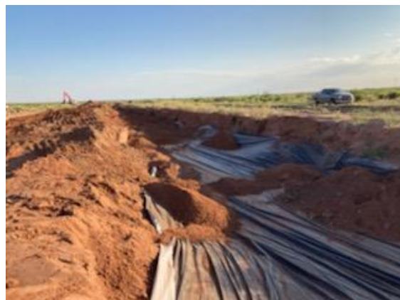
20 ML liner installed in excavation
