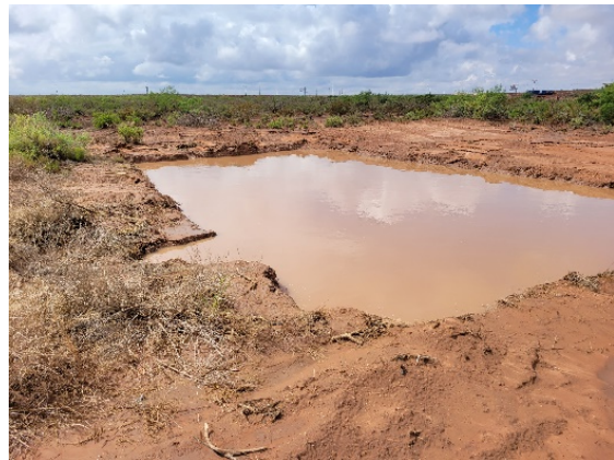
Flooded excavation due to heavy rain
