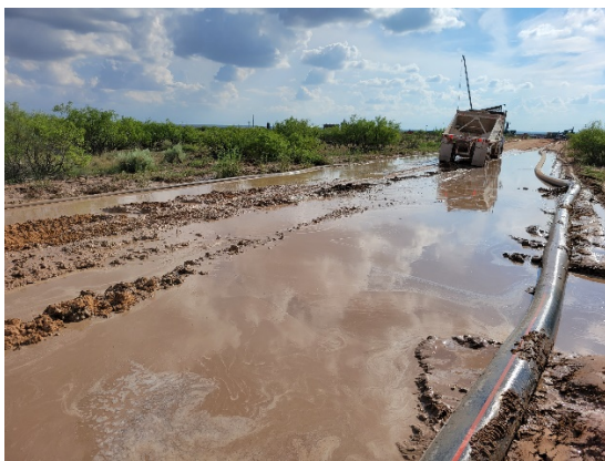
Photo of the washed out road due to Heavy rain
