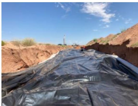
Liner properly seated in excavation
