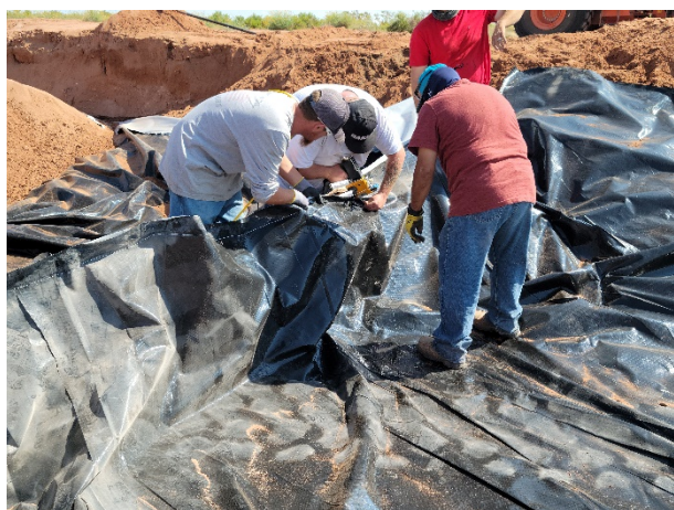
Sewing liner together in excavation
