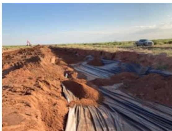
20 ML liner installed in excavation
