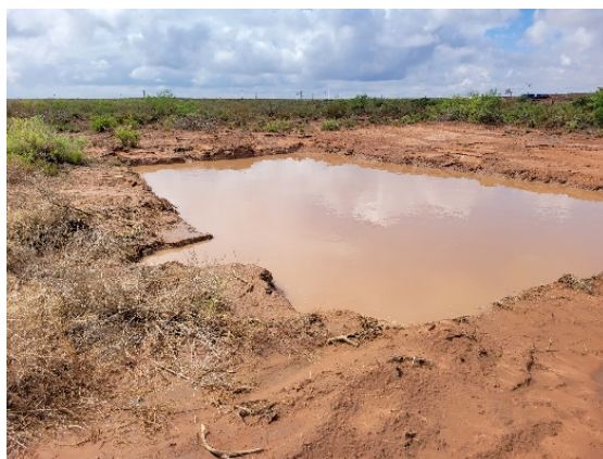
Flooded excavation due to heavy rain
