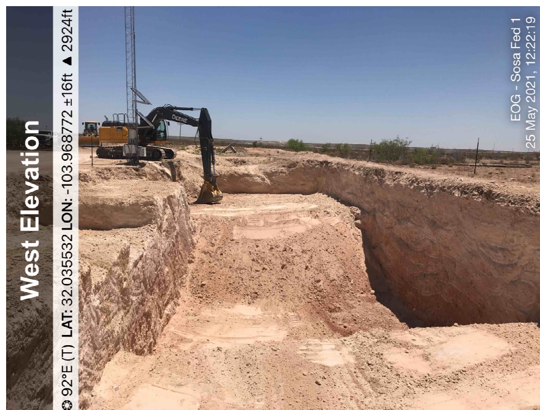
View of Release Area – View Northwest
