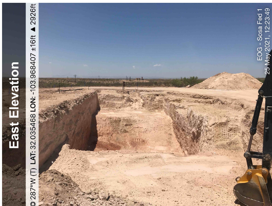
View of Remediation Activities – East View
