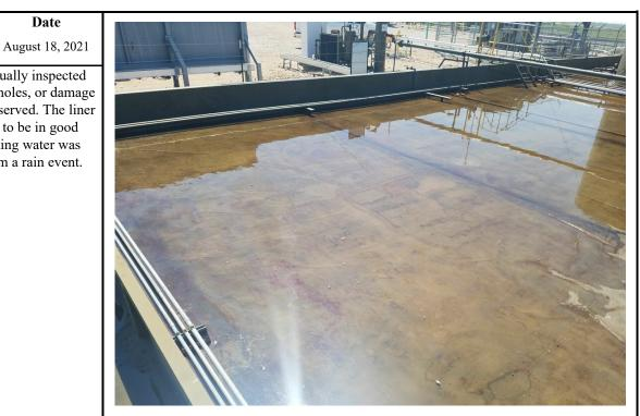
The liner was visually inspected and no rips, tears, holes, or damage in the liner was observed. The liner was determined to be in good condition. Standing water was precipitation from a rain event.
