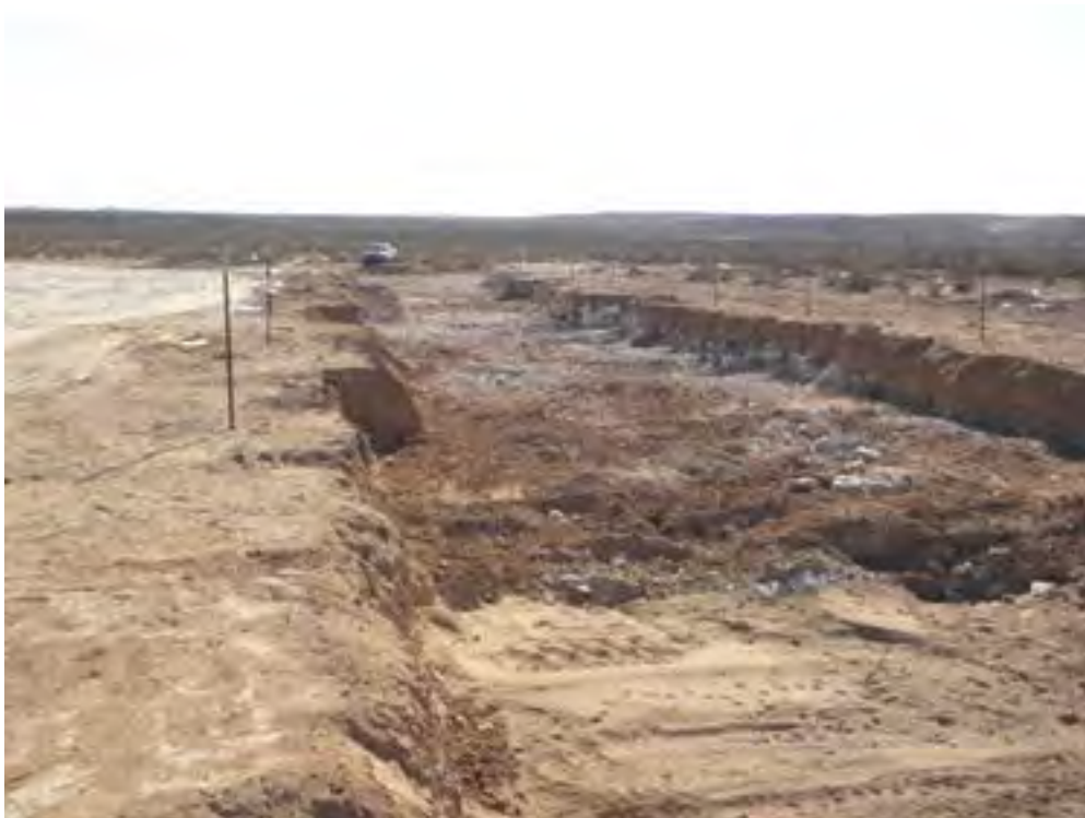
Photo 16: View of excavated area's lower region facing southeast
