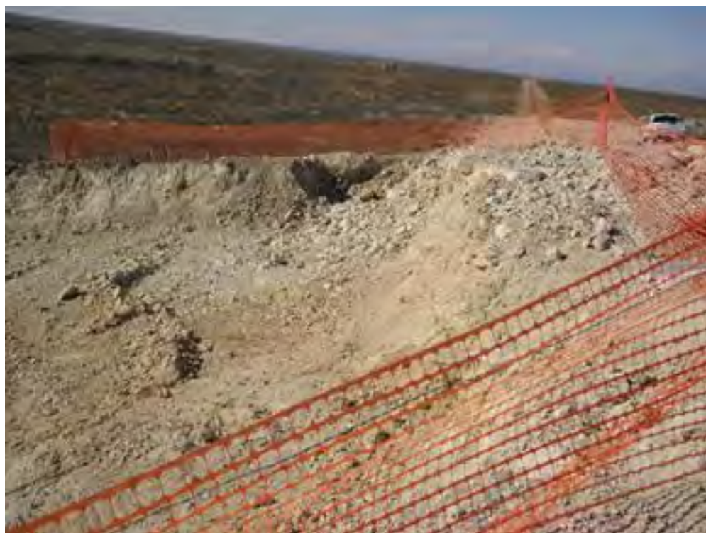
Photo 20: View of excavated area's northern boundary facing west at pipeline right-of-way
