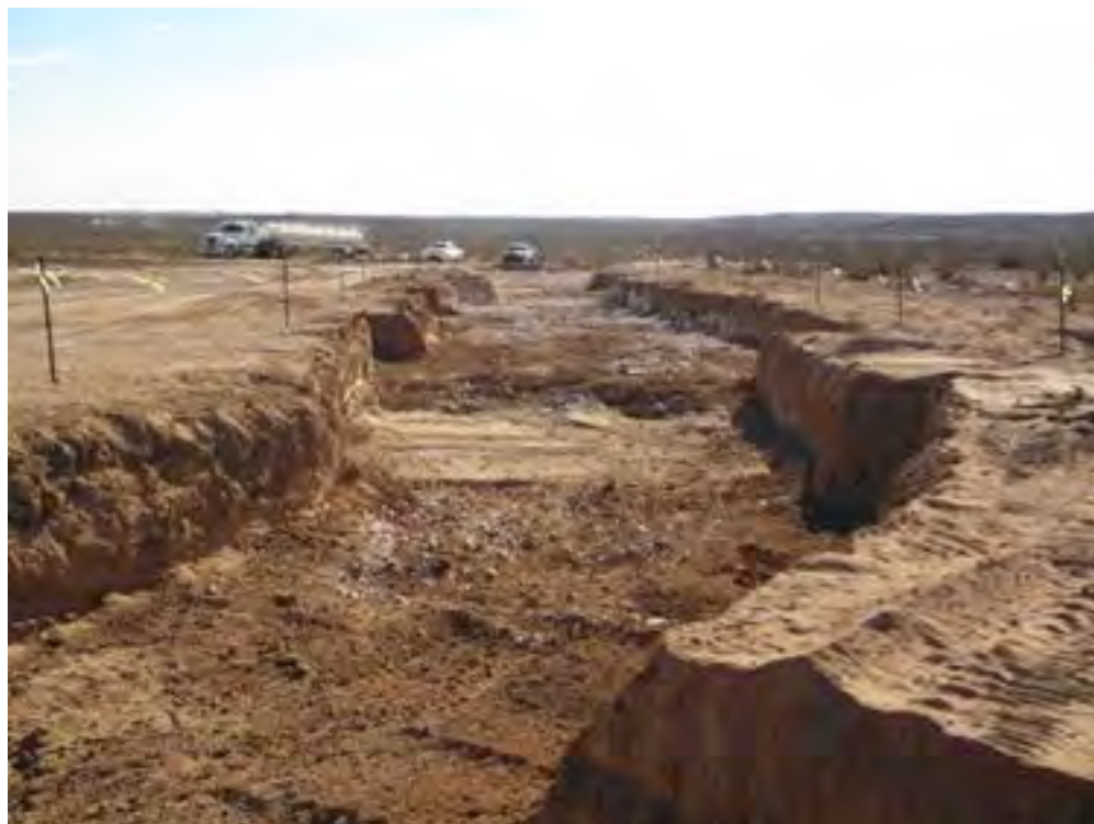
Photo 17: View of excavated area's central region facing southeast
