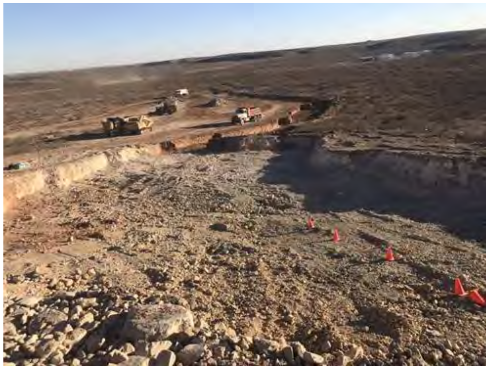
Photo 19: View of excavated area's upper region facing south from pipeline right-of-way
