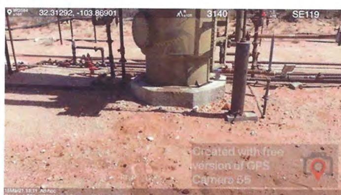
Staining from heater treater.
