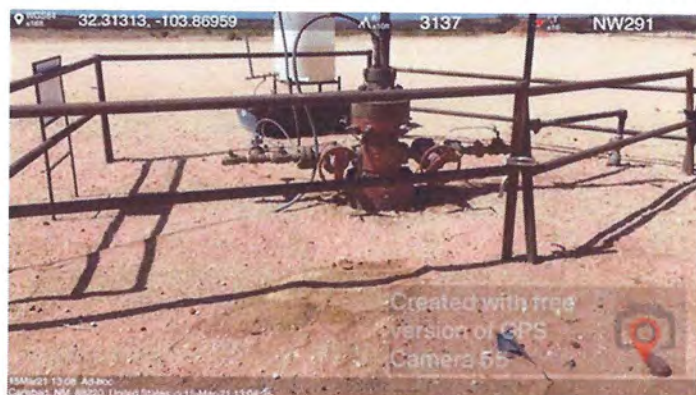
Staining around wellhead on unit #14.
