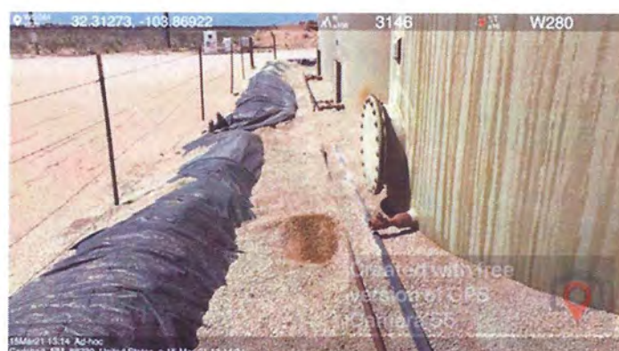
Gravel around tank battery, top layer of gravel scraped away.
