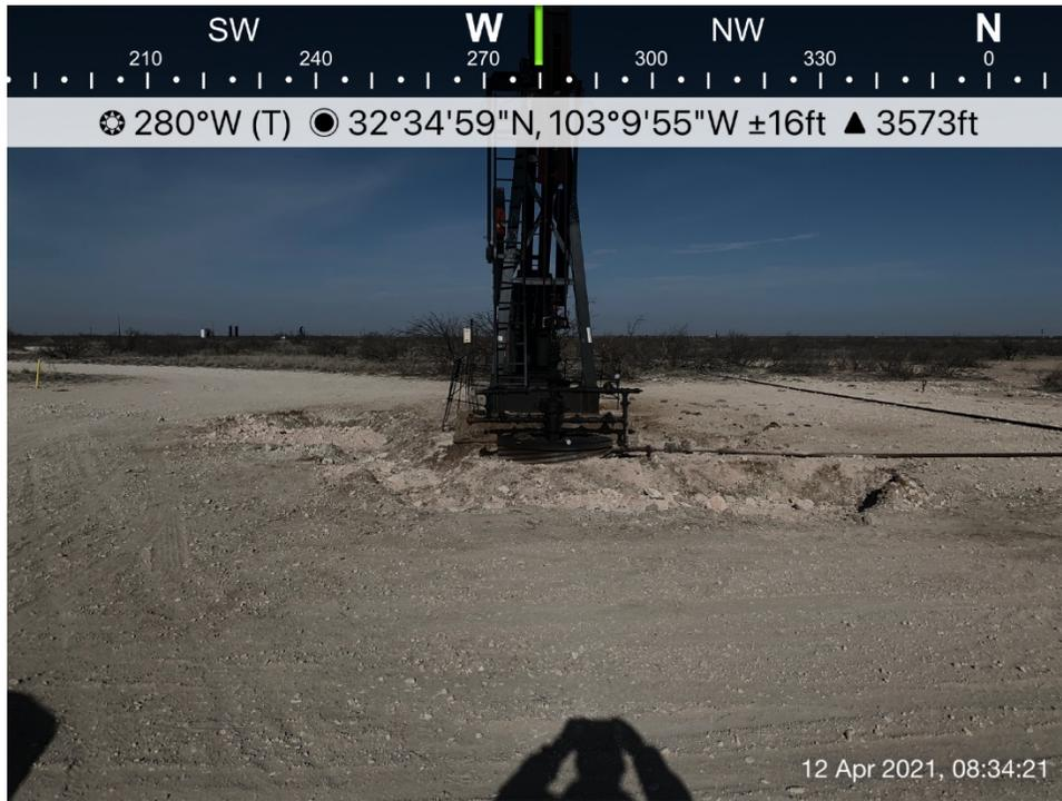
Soil Initial Excavated to a Depth of Approximately 1.5 feet bgs
