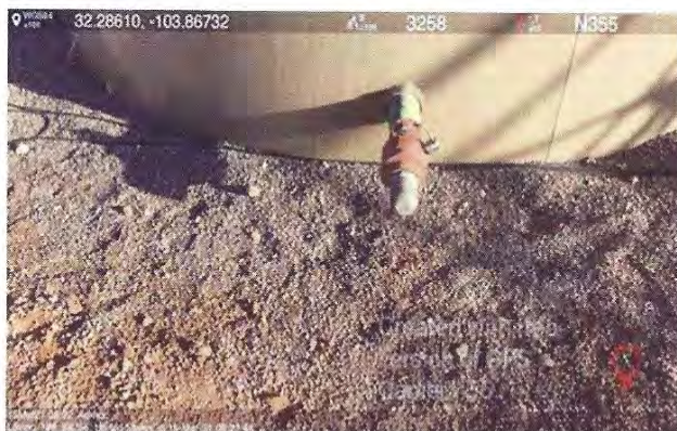
Tank drain valve with gravel with light staining.
