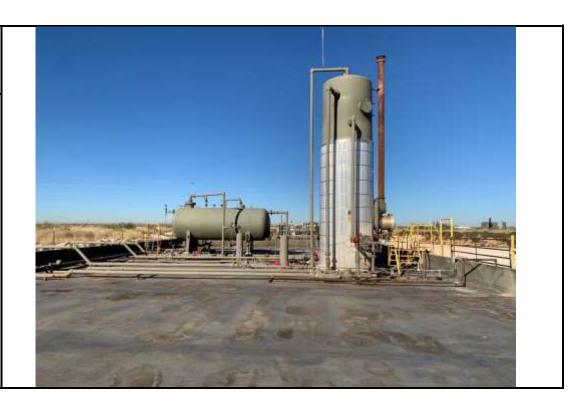
The liner was visually inspected and no rips, tears, holes, or damage in the liner was observed. The liner was determined to be in good condition.
