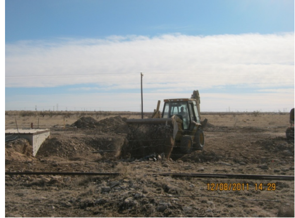
Backfilling with blended backfill, facing south 12.8.11
