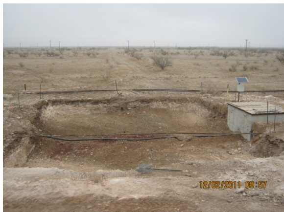
Site excavated to 49x44x5-ft deep, facing north 12.2.11
