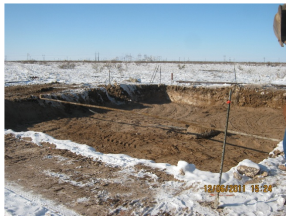
Installed bottom 6" sand pad, facing northwest 12.6.11
