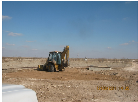
Backfilling top 6" with blow sand, facing east 12.9.11
