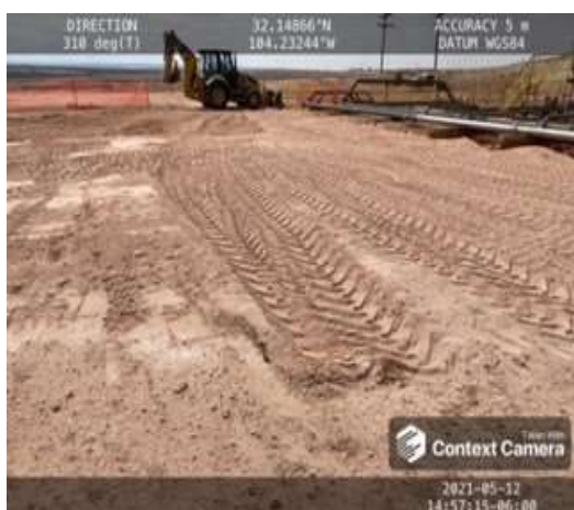
Backfilled exterior of containment to grade
