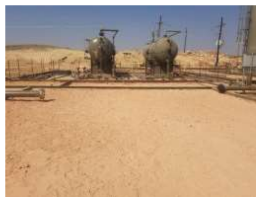
Interior of containment backfilled to grade
