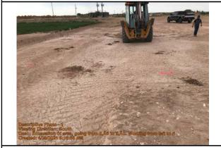
Excavation of area, going from 2' to 6". Working from left to right
