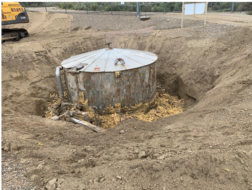
Photo 3: Aztec CDP BGT cleanup in progress
