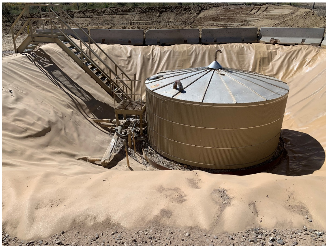
Photo 5: Aztec CDP BGT cleanup – liner installed
