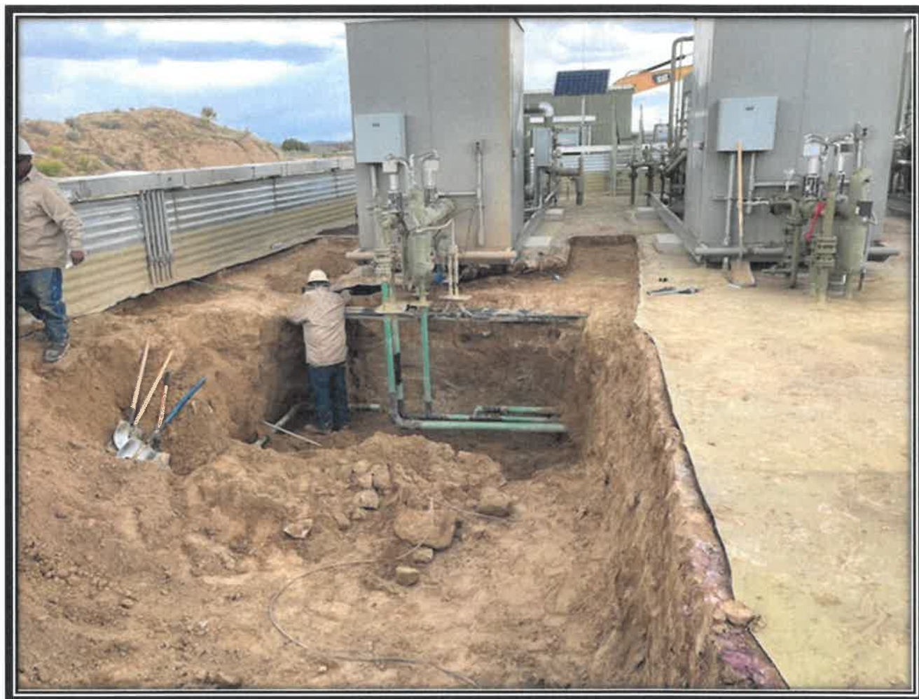
Jicarilla #103H water dump line leak.
