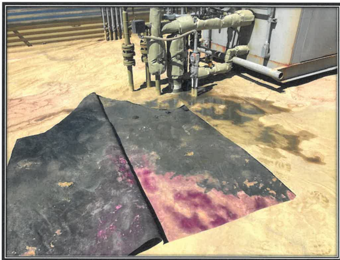
Jicarilla 103H dump line leak 8/25/2021
