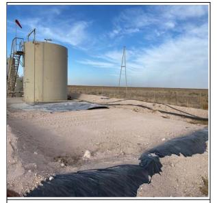
Photograph No.4 Description: Remediated area backfilled to grade
