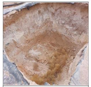
Photograph No.3 Description: Hydrovac cleaned rock shelf 13' bgs
