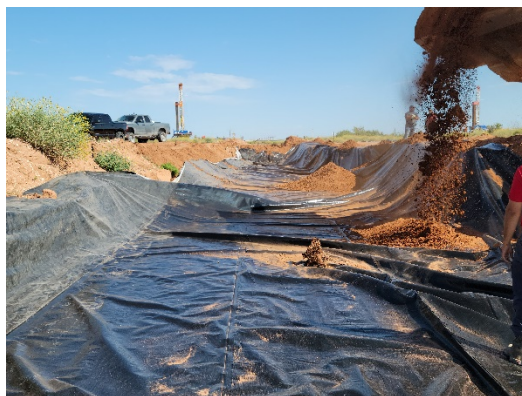
Backfilling excavation after liner installation
