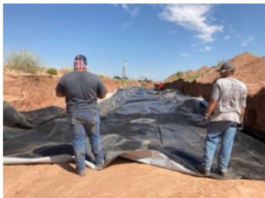
Seating liner in excavation area
