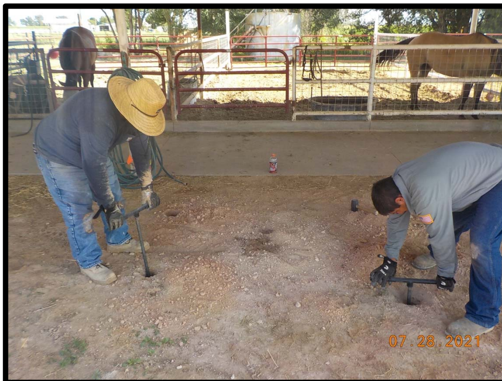
PHOTOGRAPH NO. 1 – A general view of the hand auger boring installation process during the July 2021 site assessment in the area of A-4. (Approximate GPS: 32.920392, -104.394350)
