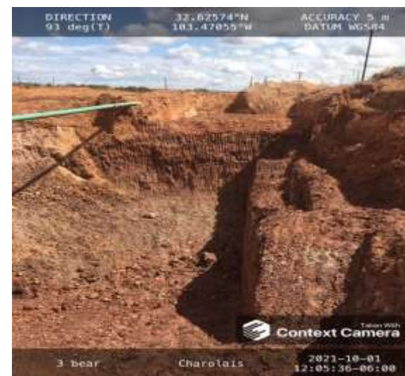
Source excavated to 25 feet bgs.
