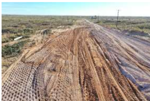
Backfilled to grade
