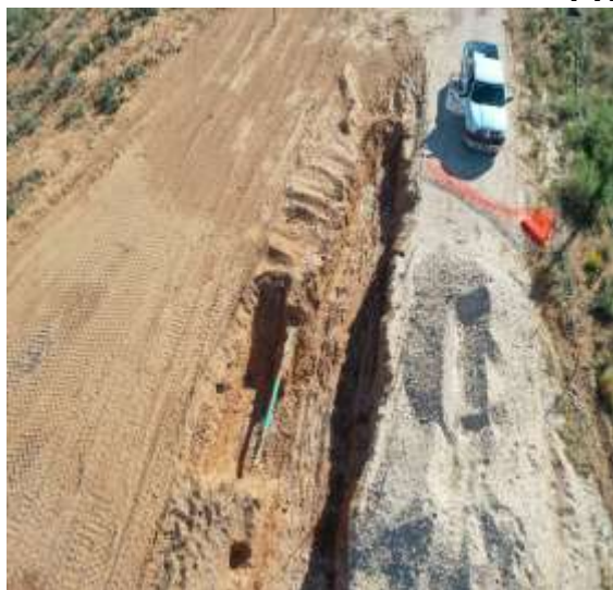
6" Line Exposed-Source and surfactant impact
