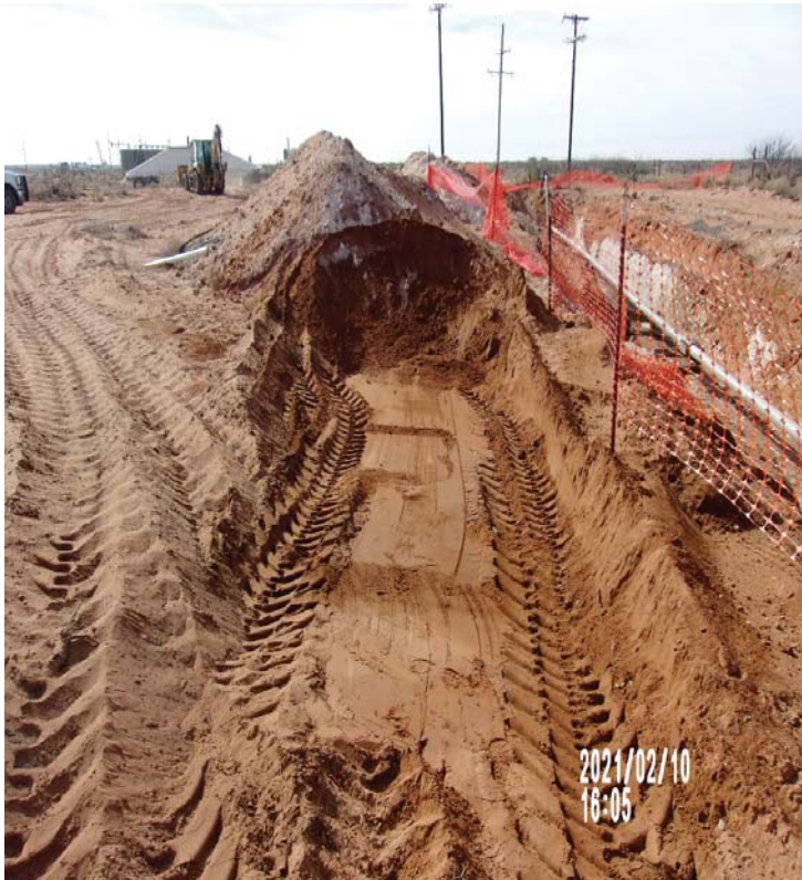
View South – Remediation (excavation of impacted material from within the release footprint) activities ongoing. Material was transported to an approved disposal facility.
