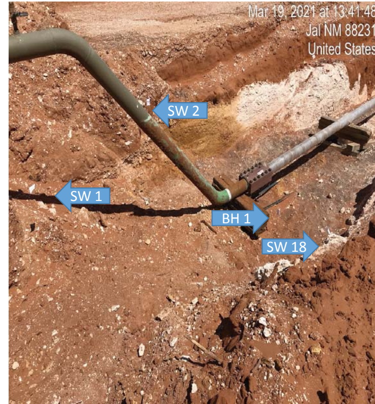
View West – Sample locations Side Wall 1 and 2, Bottom Hole 1 (7'EB), and Side Wall 18 (flagged). Blue arrows identify pin flags. Note the clamp where the repair to the pipeline was made.
