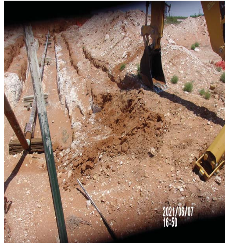
View East – Remediation activities (excavation of impacted material) ongoing adjacent to and around sample location Side Wall 18.
