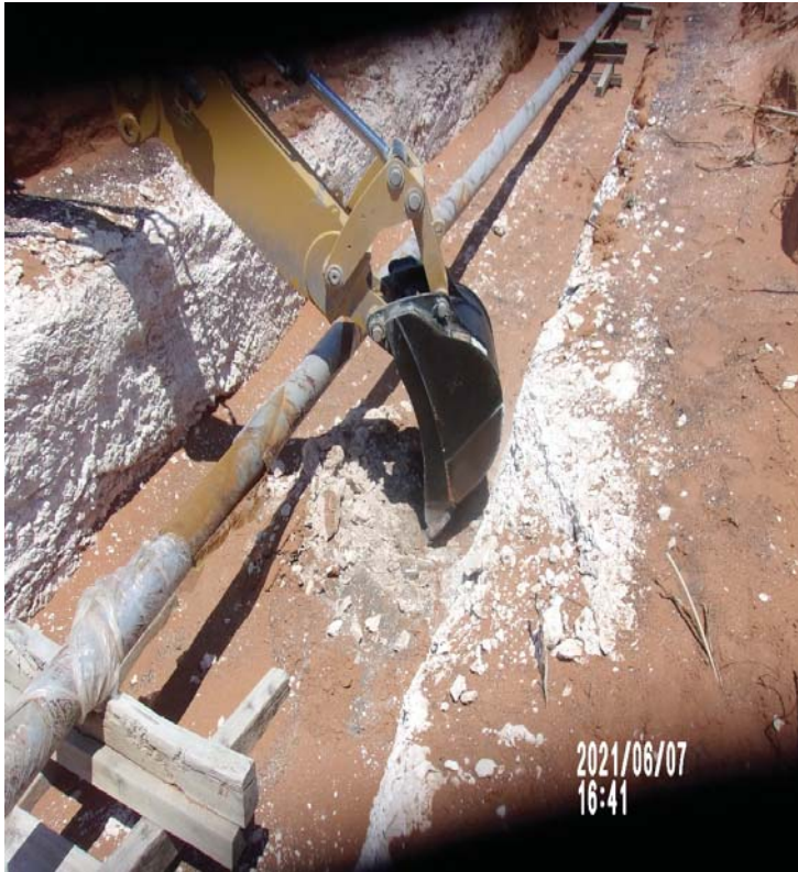
View Northeast – Remediation activities (excavation of impacted material) ongoing adjacent to and around sample location Bottom Hole 5.
