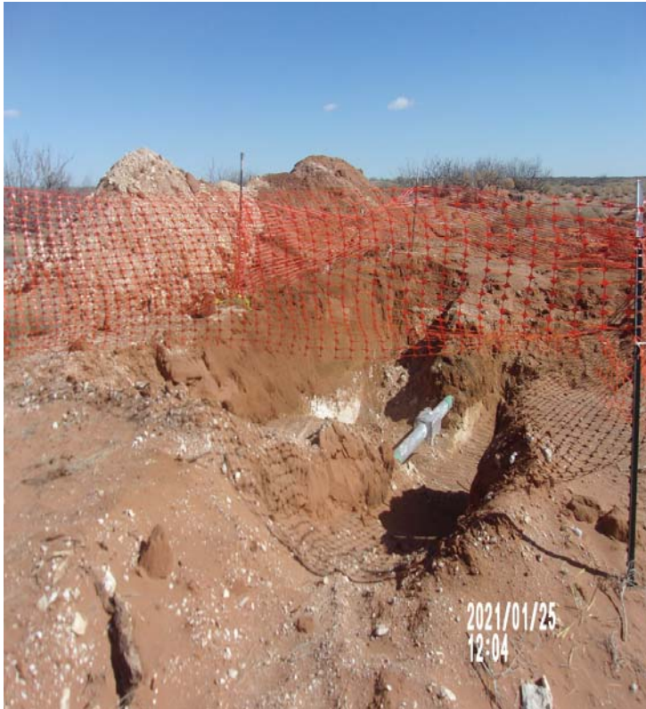
View North – Origin of spill. Cause of the release is due to corrosion on a buried pipeline. Note a portion of the spill flow path (dark brown staining) within the release footprint.
