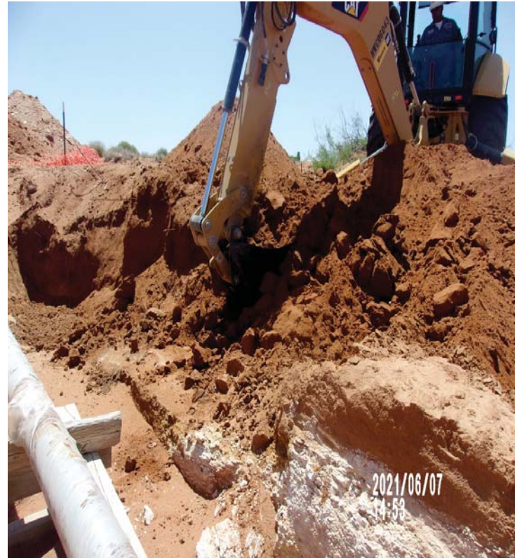
View Southeast – Remediation activities (excavation of impacted material) ongoing adjacent to and around sample location Side Wall 12.
