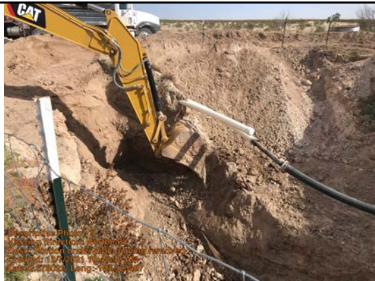
Portion under piping being removed
