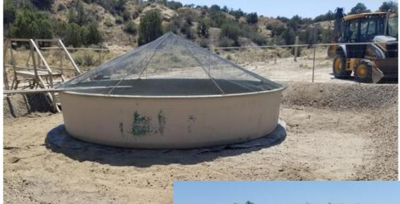
An Above Grade Tank (AGT) has been placed in the area where the BGT was previously located. The ground has been leveled up to match the contour of the site and a berm built around the AGT.
