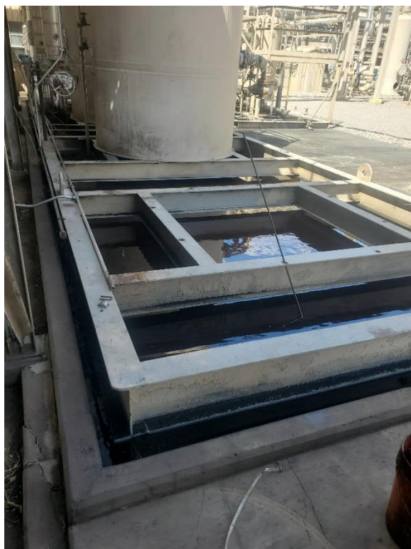
Photo 1: Amine in cement secondary containment August 23, 2021
