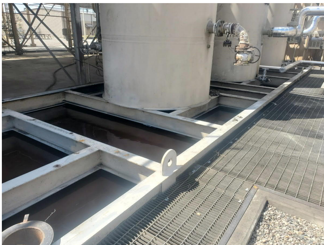
Photo 2: Amine in cement secondary containment August 23, 2021
