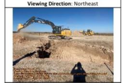
Excavation is being kept on east side as much as possible to make sure equipment can get to the pipeline when it is removed
