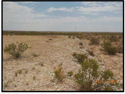
PHOTOGRAPH NO. 4 – A view of the southern pad boundary noted to be raised above the natural grade of the surrounding area. The view is towards the east.
