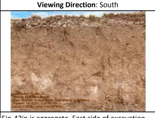
5in-42in is aggregate. East side of excavation.
