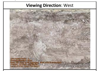
6in down to 4ft aggregate. West side of excavation
