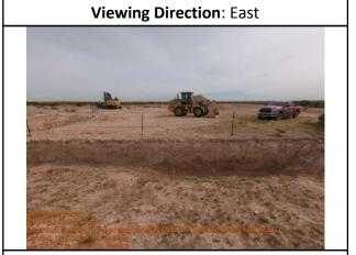
East SW 4' out from an abandoned 3" Steel line from the former we'll head is still hot. Waiting on approval by EOG to step out closer or have the line removed.
