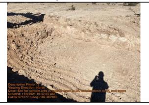
Soil for sample area is topsoil down to 2ft, caliche down to 4ft, and aggregate on the bottom
