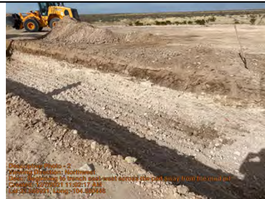
Beginning to trench east-west across the pad away from the mud pit
