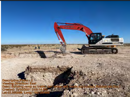
Building ramp so excavator and loader can scoop dirt inside excavation. Reason for this is pipelines on east side of the pad are in the way
