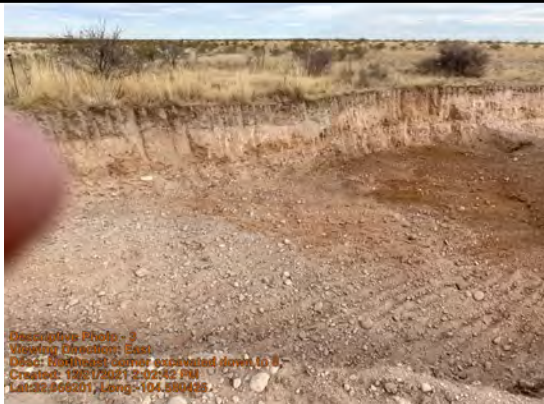
Northeast corner excavated down to 8'
