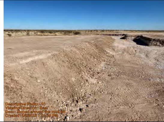
Sloped around the mud pit
