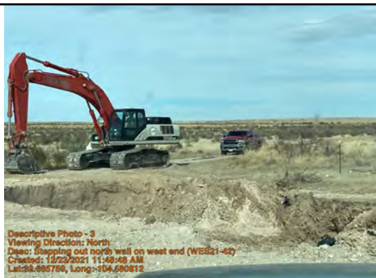
Stepping out north wall on west end (WES21-42)
