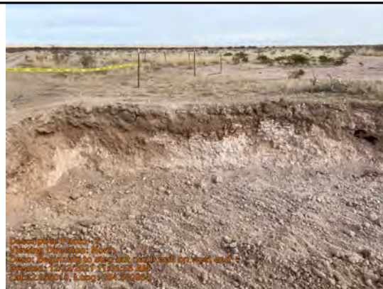
Beginning to step out north wall on west end. Not going too far to east where mud pit is
