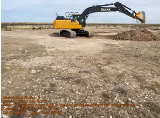
Excavating down 4' to the end of the dead spot SW of the well head
