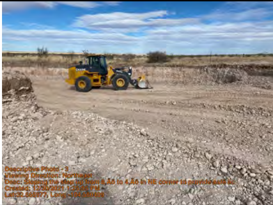
Sloping the step up from 8' to 4' in NE corner to provide safe access
