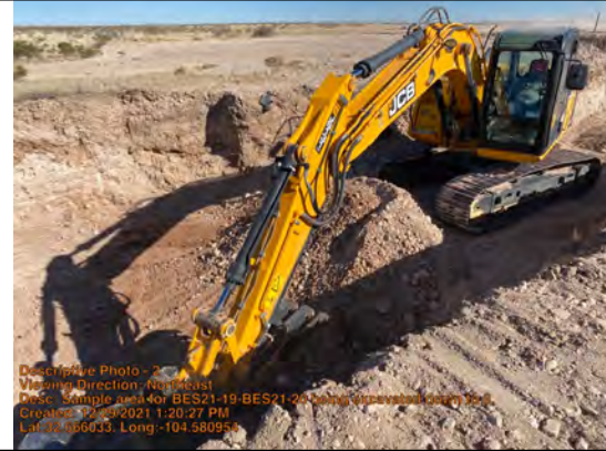
Sample area for BES21-19-BES21-20 being excavated down to 8'
