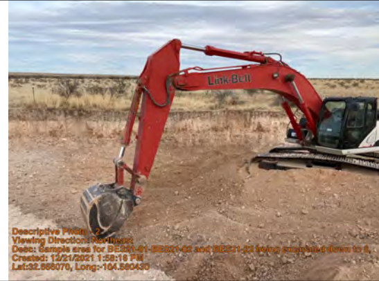
Sample area for BES21-01-BES21-02 and BES21-22 being excavated down to 8'
