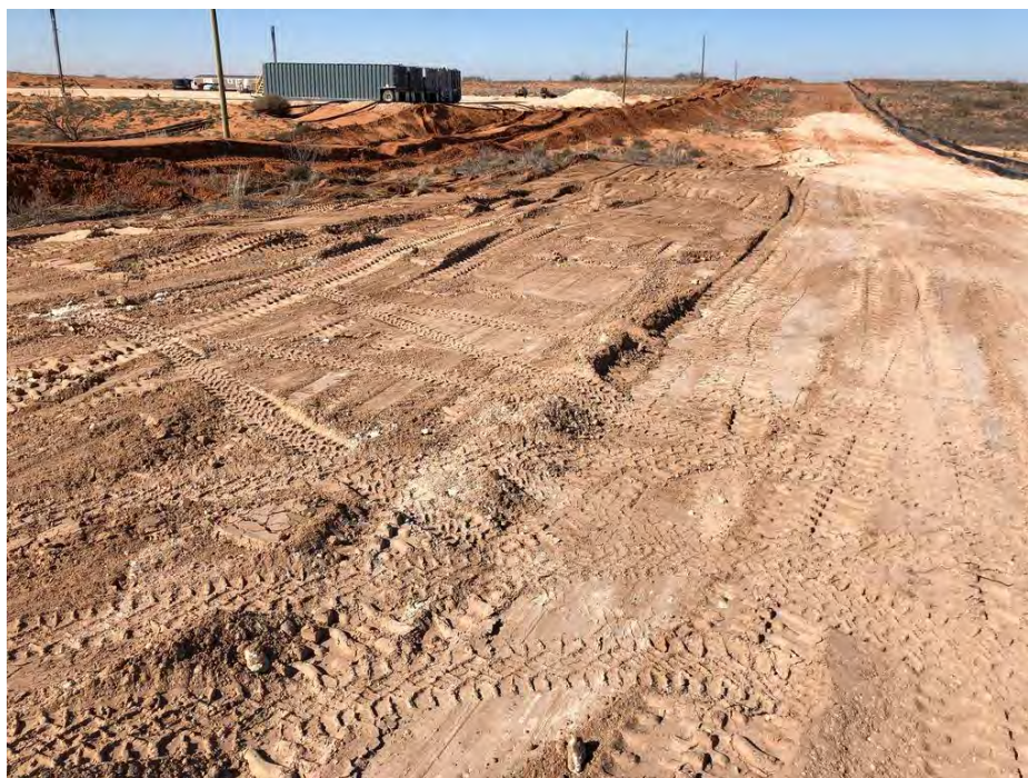
Figure 6: Backfill of release extent. Final contouring will occur during the completion of pipeline installation. The pipeline excavation is visible in photo background left. Photo is viewing north. Date: 02/14/2020. GPS: 32.4515417 N, 103.6040278 W
