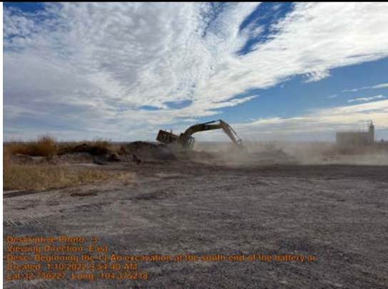
Beginning the 14' excavation at the south end of the battery area
