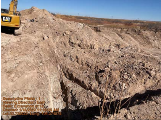
Excavation at 16' with an 18' sampling trench
