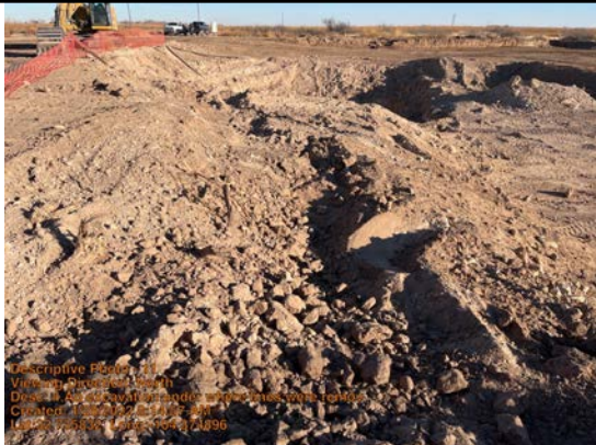
4' excavation under where lines were removed
