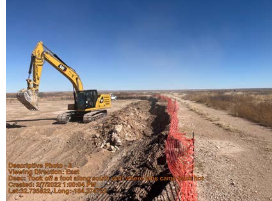
Took off a foot along south wall where labs came back hot
