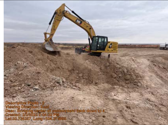
Bringing center of containment back down to 4'
