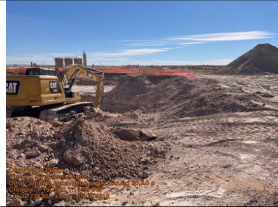
Sloping excavation sides around 20' pit
