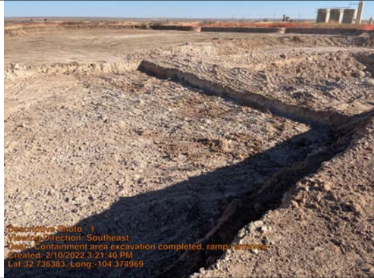
Containment area excavation completed, ramp removed
