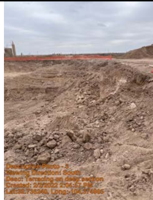
Terracing on deep section
